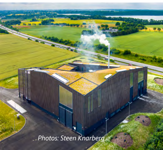
Left: The 12 MWth / 1MWe cogeneration Sorø Bioenergy plant. Middle: The gasification furnace can use a mix of difficult fuels such as garden-parc biomass. Right: The top of the Dall Energy gasification furnace in Sorø
