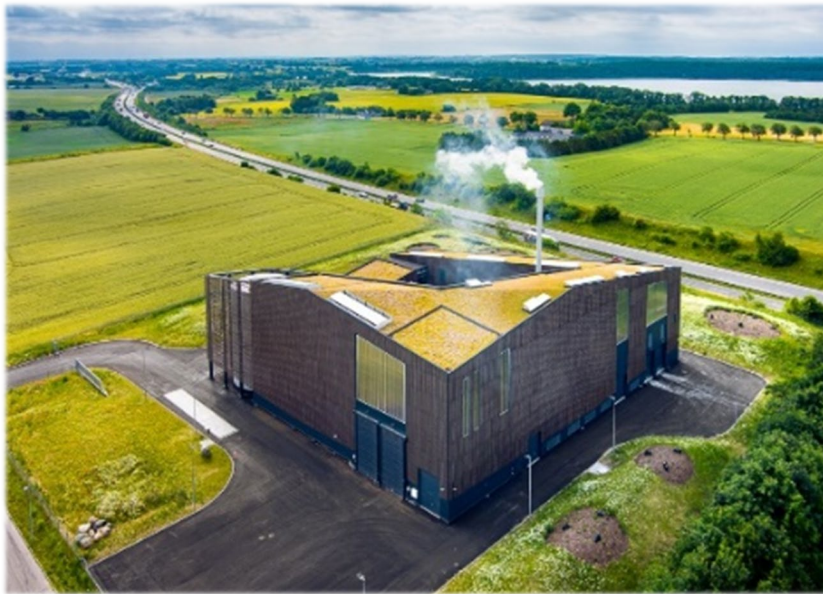
Sorø cogeneration plant 2021, 12 MWth/1MWe
