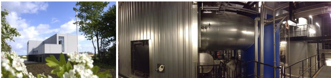
Figure 42: 9 MW Dall Energy plant in Sønderborg
