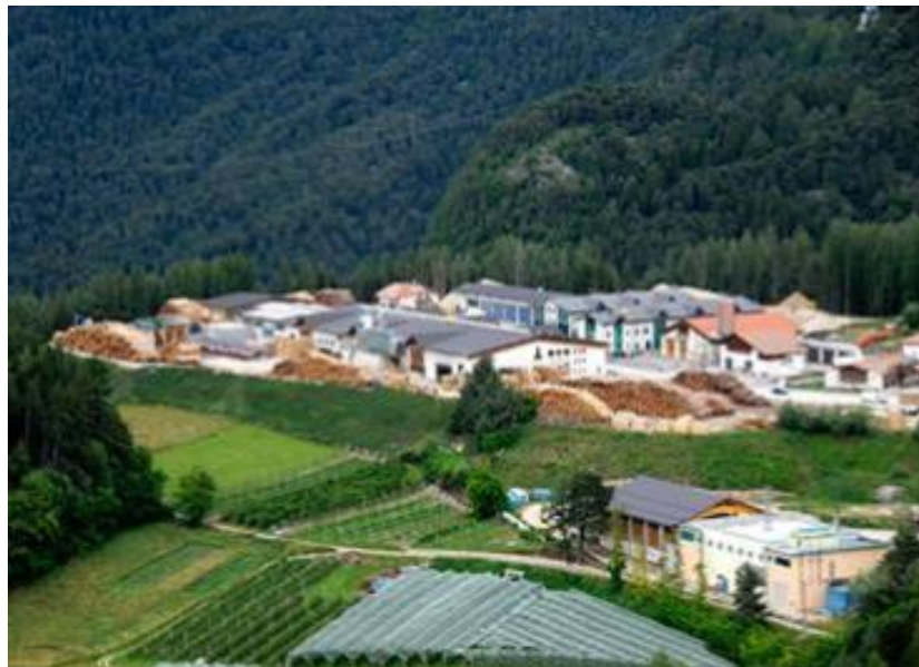
Figure 25: CHP plant in Fondo, Italy (by courtesy of Heliex Power Ltd)
