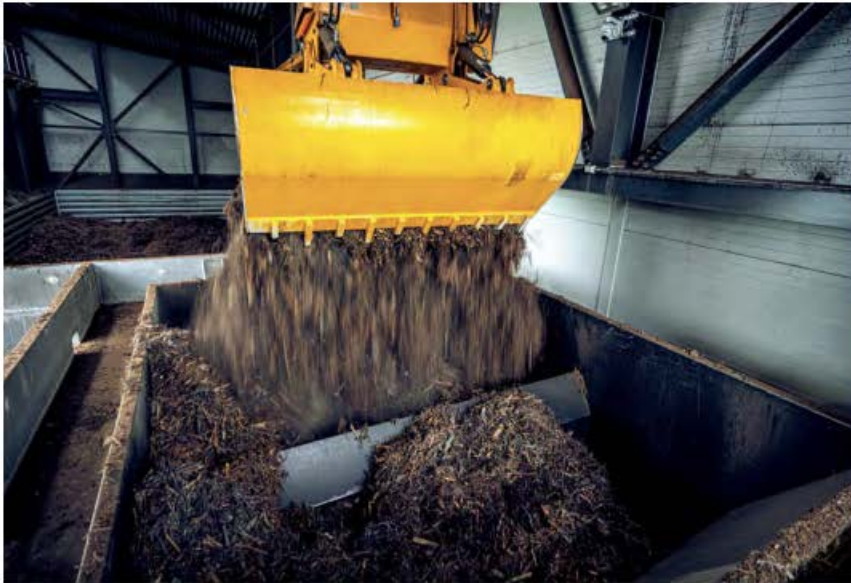
Dall can process locally sourced biomass
