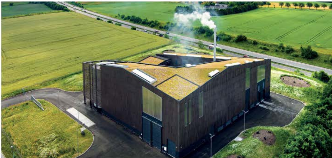
Sore, Denmark plant
